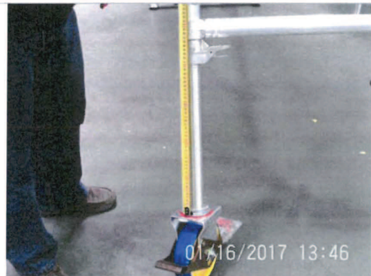
50. Screwjacks measure (extended part)
